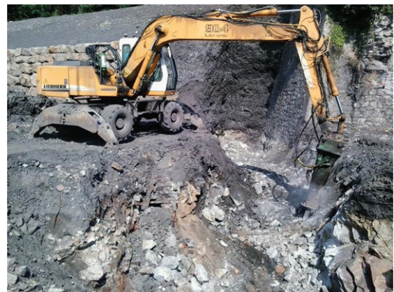
Fig. 2. Wheel excavator operator working with a rock breaker for foundations preparation.
