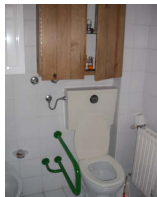
Fig.5: Bathroom - 2 nd floor Home for the Elderly.
