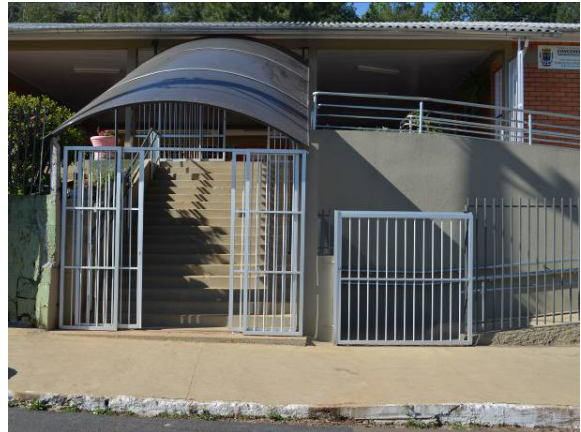
Figure 4: School Access – ramp access closed
