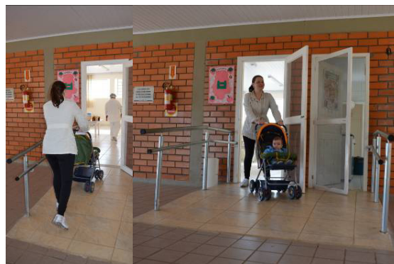
Figure 8a e 8b: Mother access the refectory without difficulties. Ramp with handrails in two heights
