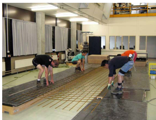
Figure 1. Four ironworkers lifting a 100-kg lattice
