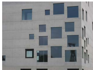
Fig. 3 – Design School Essen, a concrete construction with integrated active insulation.
