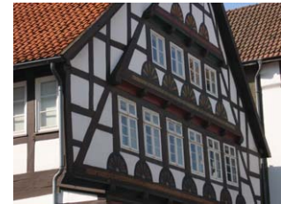
Fig. 1 – Timber frame construction with clay infills.
