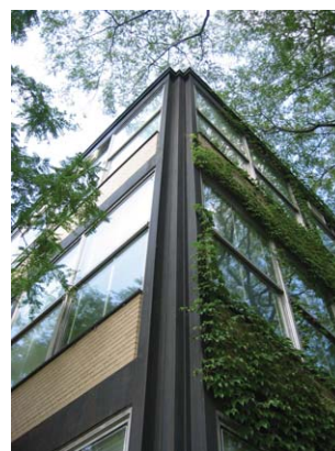
Fig. 8 – IIT Campus building in Chicago with the typical Mies van der Rohe corner solution.
