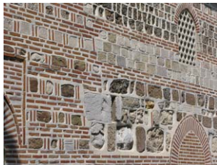
Fig. 2 – Mixed natural stone and burned clay brick masonry.
