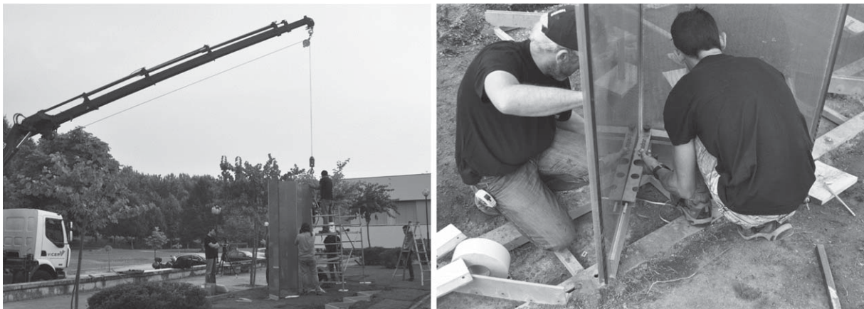
Fig. 15. Placement of the panels in position, using a crane (left) and verification of the angle between panels (right).
