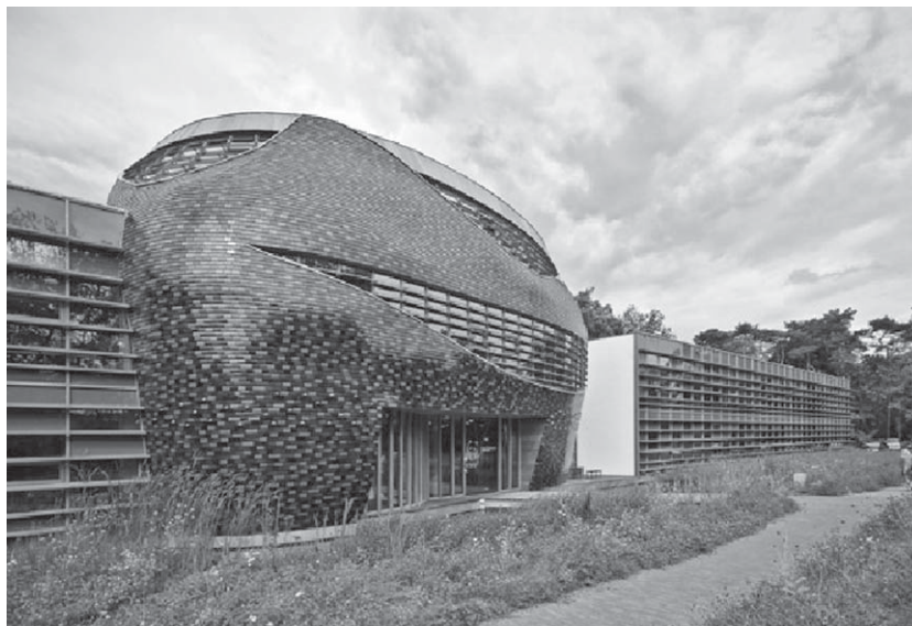
Fig. 3. Impression of the selected façade renovation solution of the WNF office building (source: vd Meijden).
