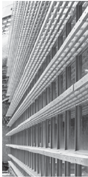
Fig. 15. Picture of the realized WNF façade renovation (source: vd Meijden).
