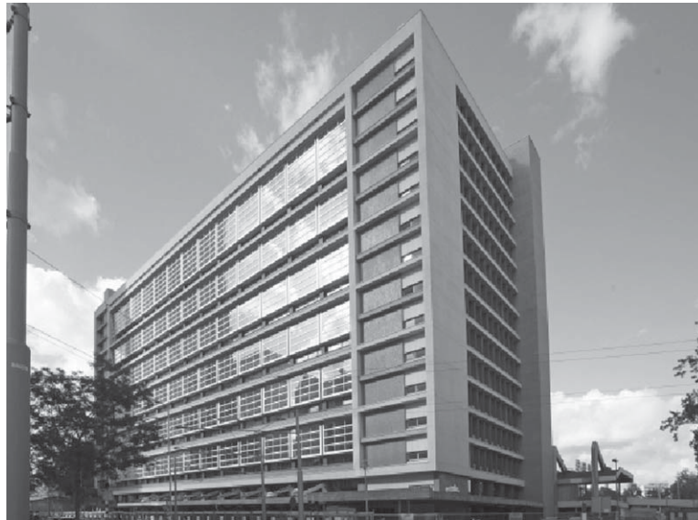
Fig. 4. Impression of the selected façade renovation solution of the Central Post office building (source: vd Meijden).
