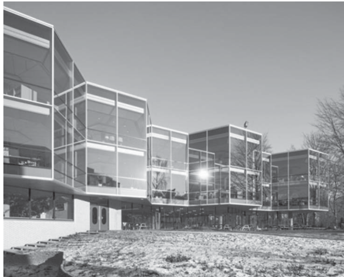
Fig. 2. Impression of the selected façade renovation solution of the DHV office building (source: vd Meijden).
