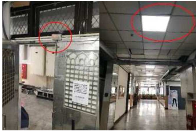
Fig. 6. bNode set on the ceiling or the door.
