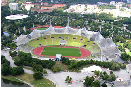
Fig. 12. The roof tensile structures by Frei Otto of the Olympiapark, Munich, 1972. Foto: Dave Morris from Edinburgh, UK.
