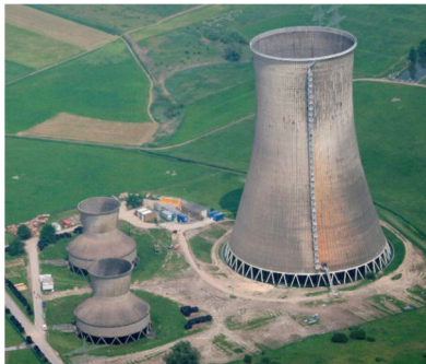
Fig. 18. Ventilation cooling towers (forced draft) and natural draft cooling tower located at power station Westfalen. Replacing part of the cylindrical surface with a minimal one increases the wind resistance of the tower.
