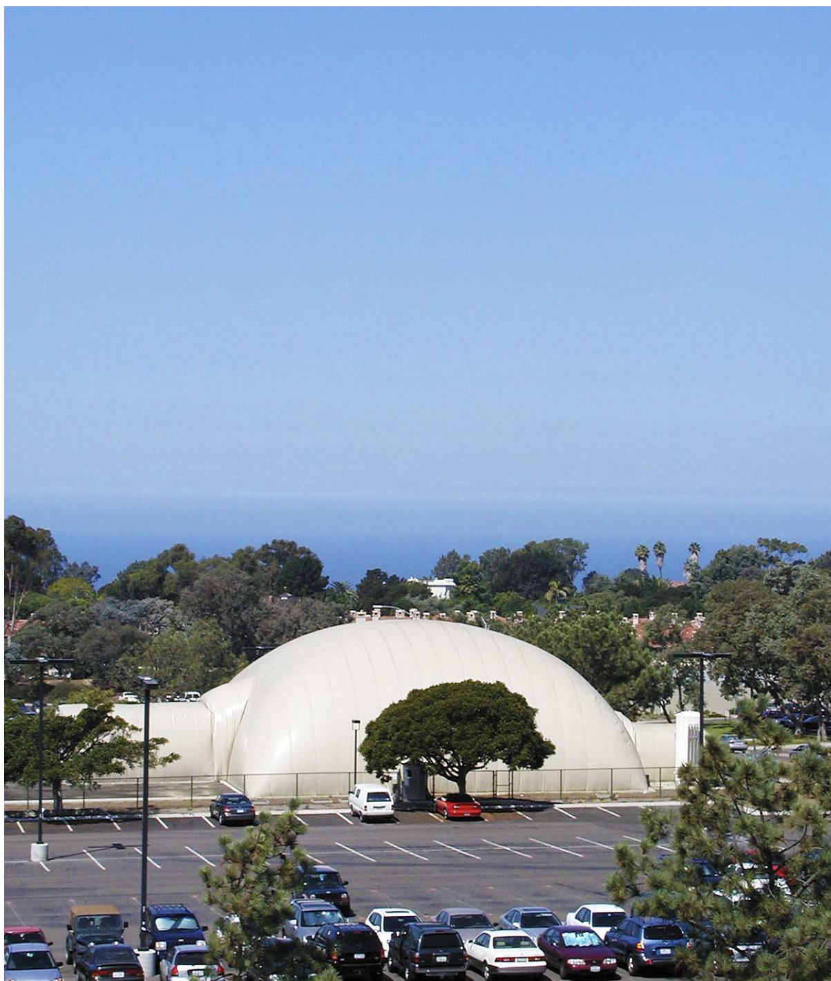
Fig. 3. The NMR spectrometers which Stanley Opella's group operate are housed in this air-supported structure that is called " The Bubble ". Picture taken by Christopher Grant. (Colors are visible in the online version of the article; http://dx.doi.org/10.3233/BSI-140087 .)
